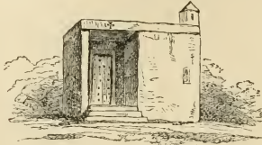
Hut of a Greek peasant formed of mud imbedding sticks and straw. (From Fellowes's Lycia .)
